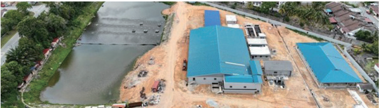
Design and Build for the Construction of New Sewerage Treatment Plant to Headwork of 36,000 PE and Upgrading of Existing Pumping Station to Headwork of 10,500 PE on Lot 13325 and Lot 17000 at Pekan Bukit Kepayang, Daerah Seremban, Negeri Sembilan Darul Khusus (Section 2)
