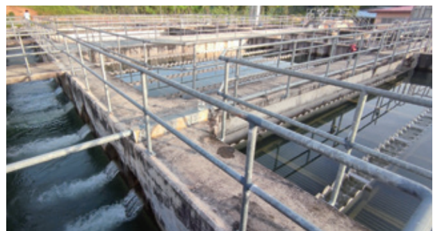
N024-P1 The Proposed Extension of Phase 2 Sawah Raja Water Treatment Plant and Other Related Works (10MGD), Negeri Sembilan. Pakej 1 – Cadangan Membina Dan Menyiapkan Loji Rawatan Air Sawah Raja Fasa 2
